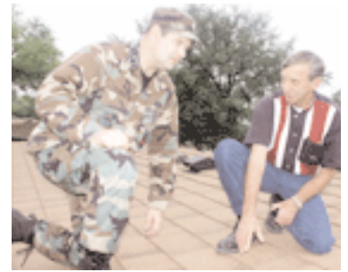
Donald Hendrix, 47th Civil Engineer Squadron construction representative, discusses a metal roof with Lt. Col. Michael Blaylock, 47th CES commander, atop a home in base housing. Mr. Hendrix earned an award of $3,969 for his idea to replace asphalt roofs with metal roofs. (photo by Tech. Sgt. Anthony Hill)
