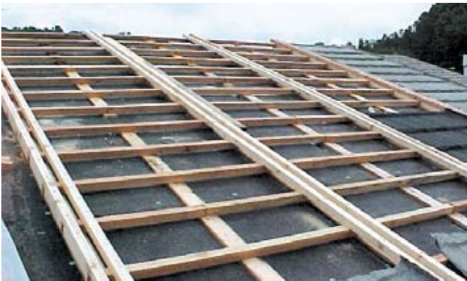
Figure 1: Batten and counter-batten system used to mount stone-coated metal roofs.
